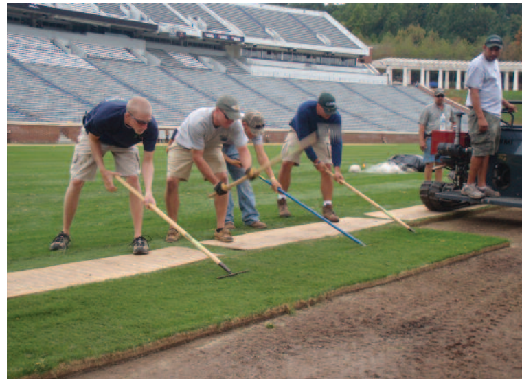
▲ Replacing the turf at the University of Virginia's David A. Harrison III Field at Scott Stadium.
